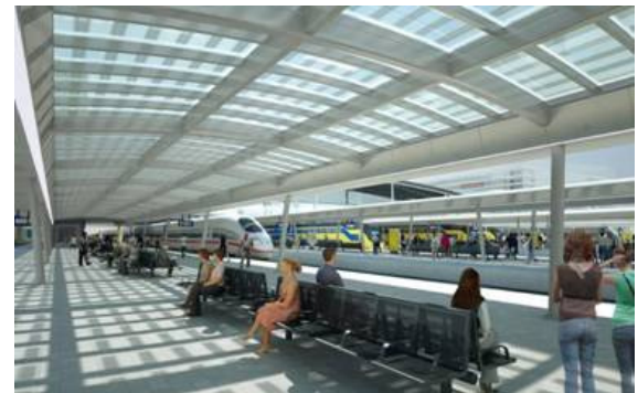
Figure 6: Impression of the station platform with transparent PV panels in the canopy above the platform (darker areas are solar cells).
