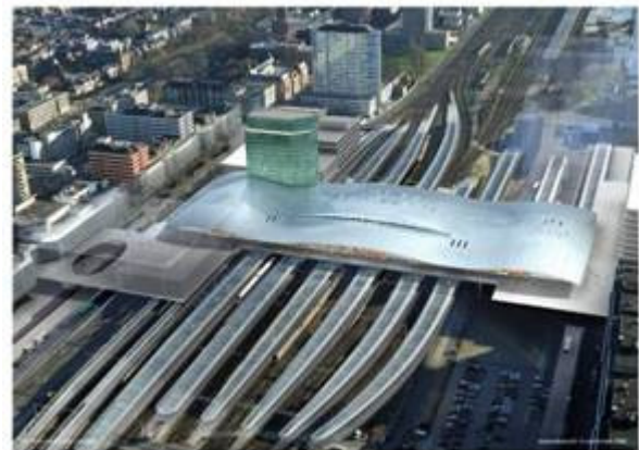
Figure 2: Artist impression of new train station. PV may be installed on the terminal roof and platform canopies.
